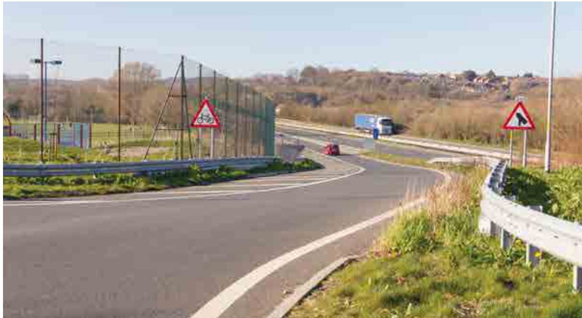
Figure 1.2 A2 London Bound On-Slip Road
